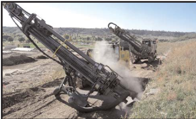
Anchor drilling in process.
