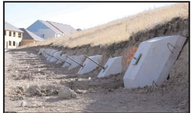
Patterned ground anchors.
